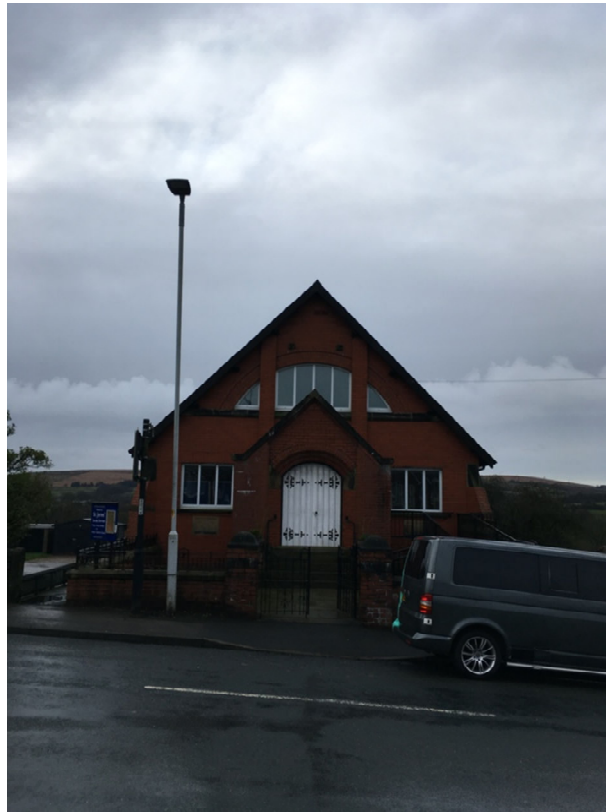
Photograph 1: St. James Mission Church External View
