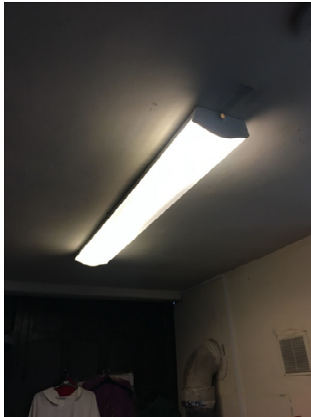
Photograph 10: Twin Fluorescent Tube
