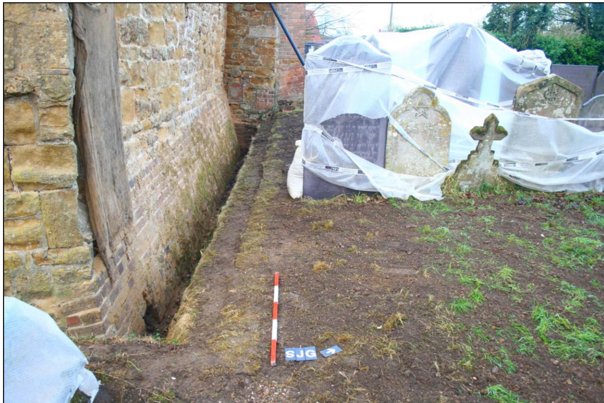
Plate 12: Completed east – west section of drain run. Scale: 1 x 1m.
