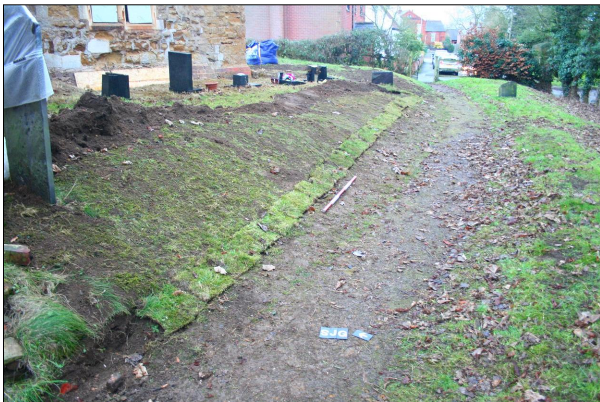
Plate 10: Completed east – west drain run. Scale: 1 x 1m.
