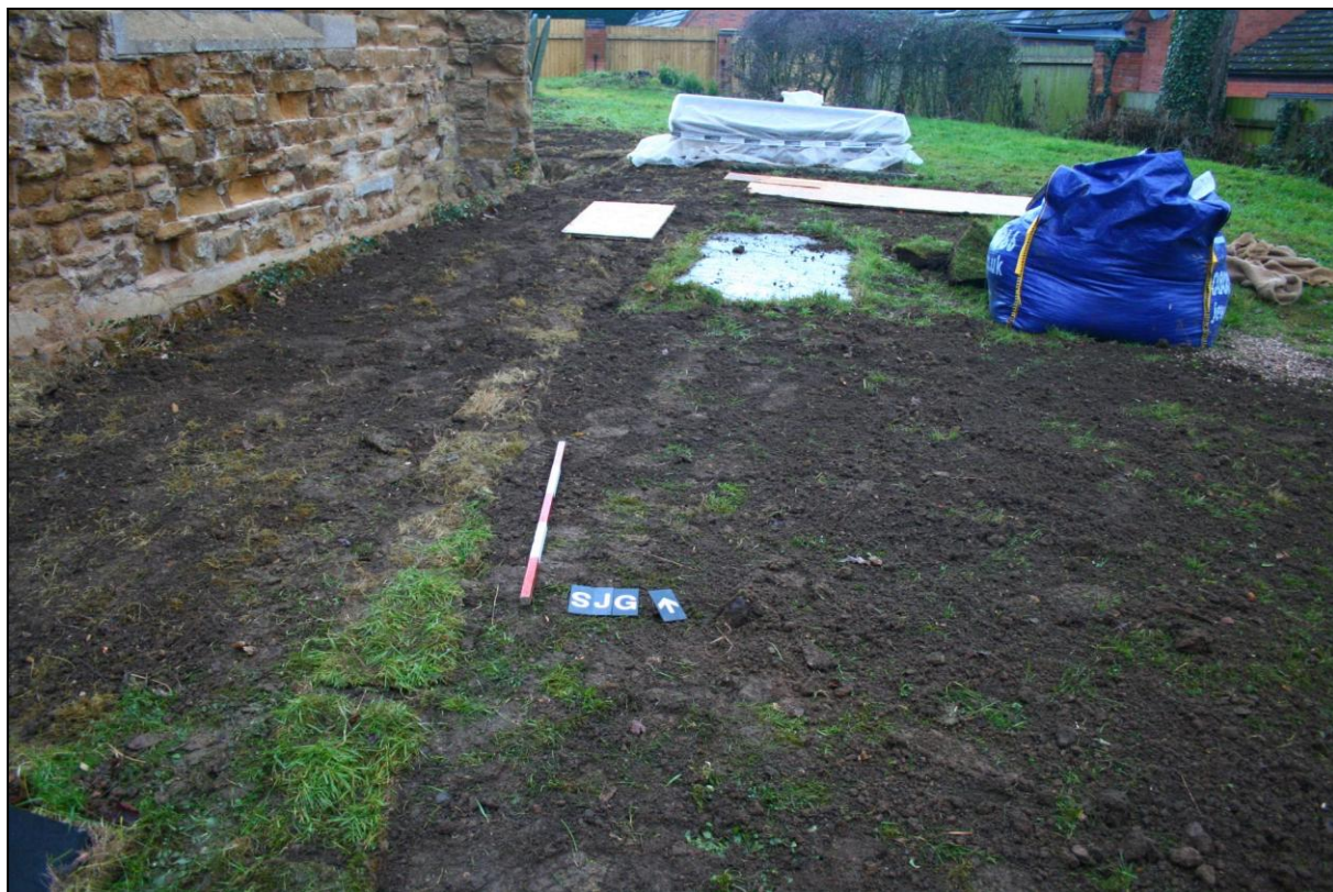
Plate 11: Completed north – south section of drain run. Scale: 1 x 1m.
