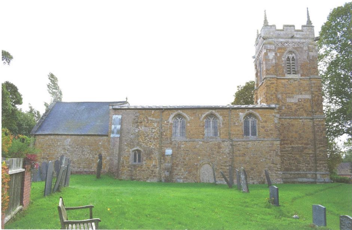
Plate 1 : General view of the church from the north.
