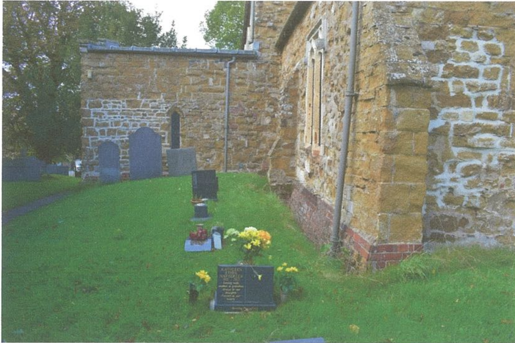
Plate 4 : View of the east wall of the south transept, looking along the south wall of the chancel.
