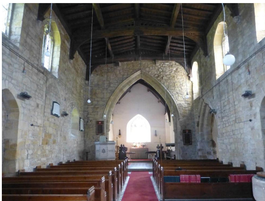
Photograph 4: Interior of nave and chancel arch
