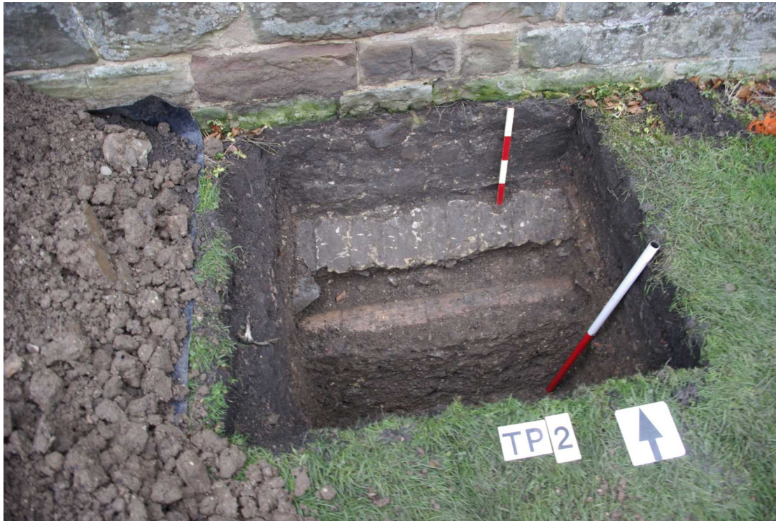
Figure 9 Test Pit 02 fully excavated 0.4m scale is resting on the angled slates laid to deflect water towards the drain
