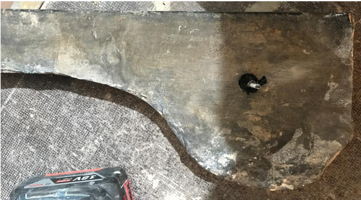
Plate 7: Supporting dowel to the back of the scroll bracket
