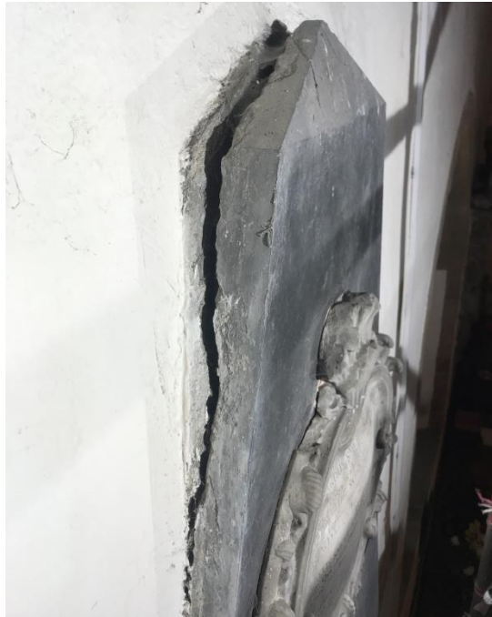
Plate 2: The gap between the upper section of the obelisk and the wall.
