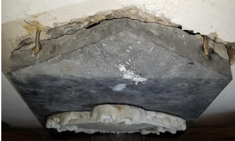
Plate 6: Fixings holding the top section of the obelisk into the wall
