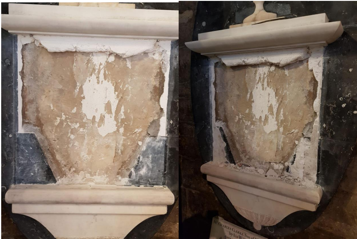
Figure 22: Image showing the deconstruction of the Clarke monument.
