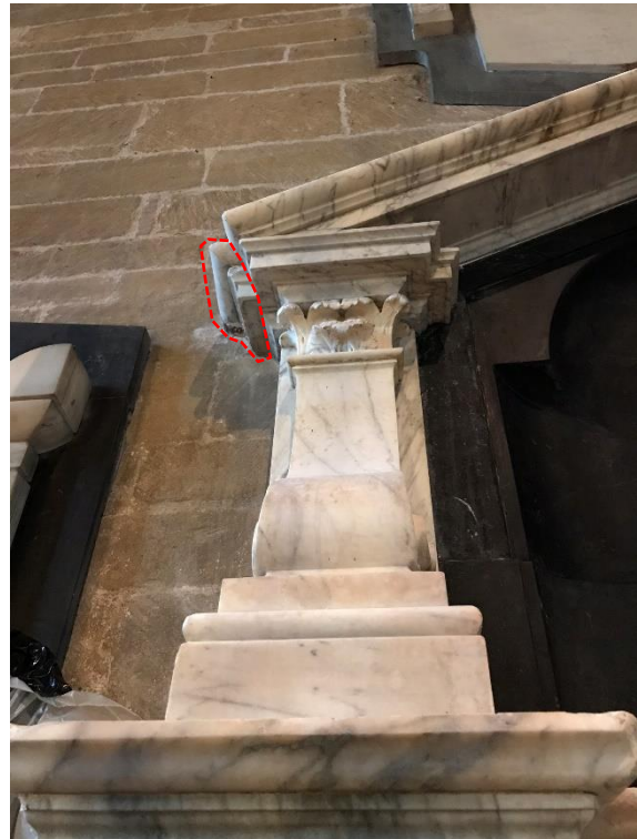
Figure 15: Section of repair with fine casting plaster.
