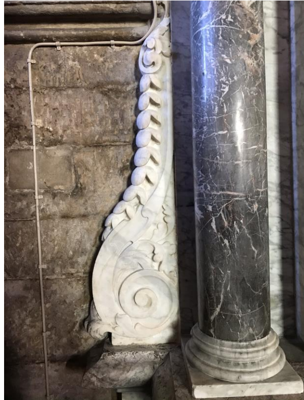
Figure 19: Post treatment condition of the decorative scrolls on the Bury monument.
