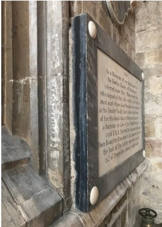
Figure 3: Plaster repairs to the side of the Newton monument.
