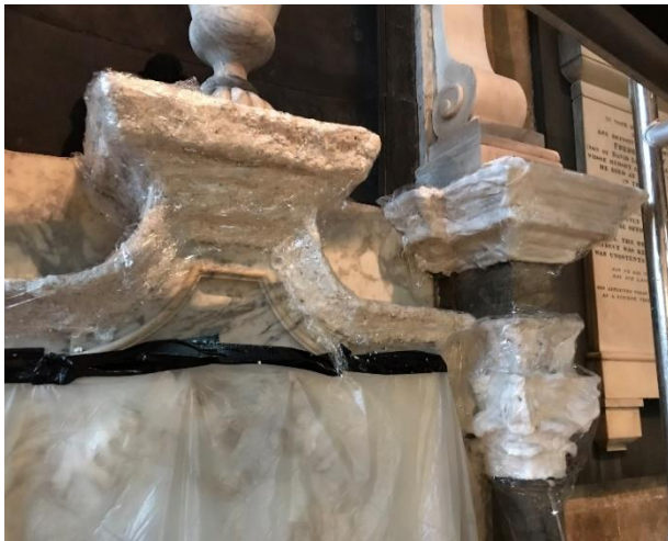
Figure 14: Image of the application of the poultice pack to the Thomas Bury monument.
