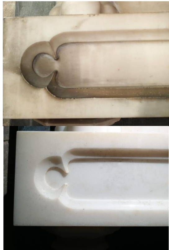
Figure 11: White marble before and after cleaning.
