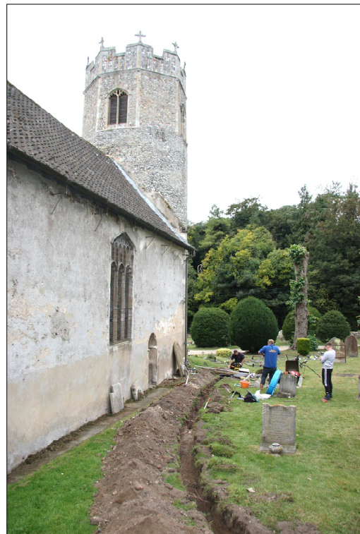
Plate 2. Trenching works in progress, looking West.
