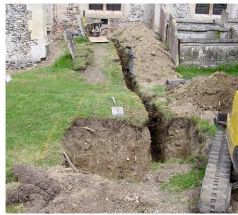
Fig. 4 Soakaway 3 after excavation, showing drain run
