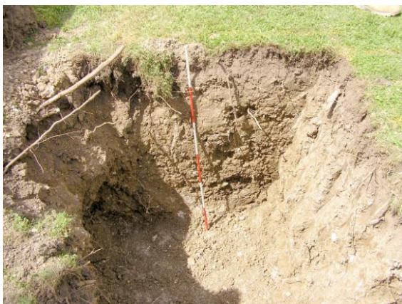
Fig. 3 Soakaway 3 after excavation, range rod totals 1.5m
