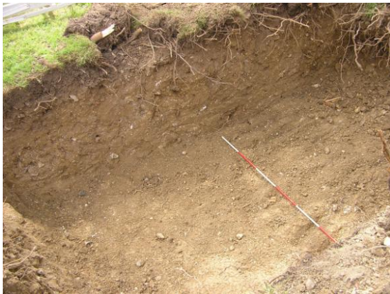
Fig. 1 Soakaway 1&2 after excavation, range rod totals 1.5m
