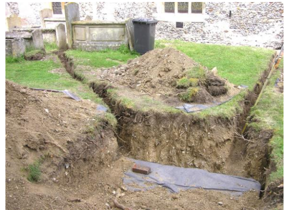
Fig. 2 Soakaway 1&2 after excavation, showing drain runs
