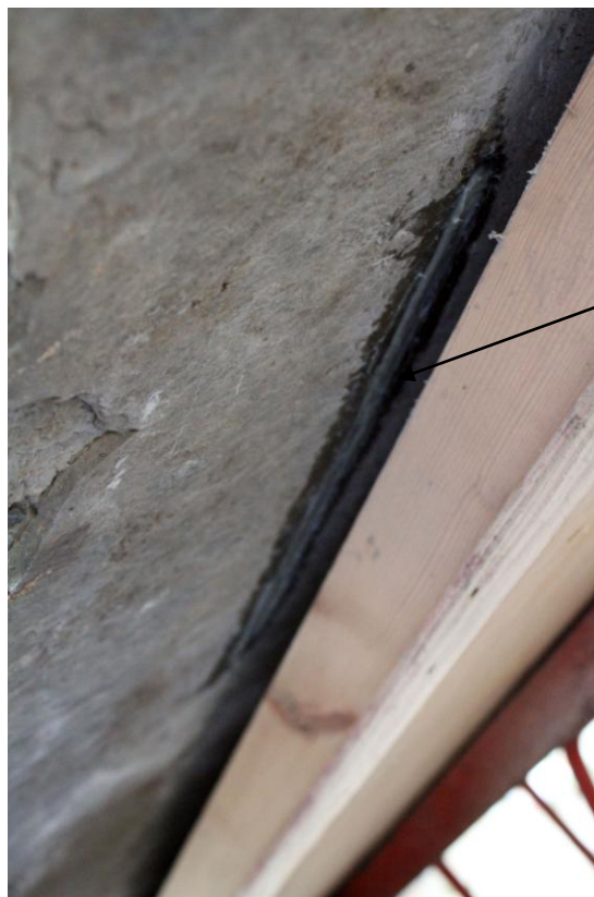
22. Rod inserted in the underside of the slab to repair crack
