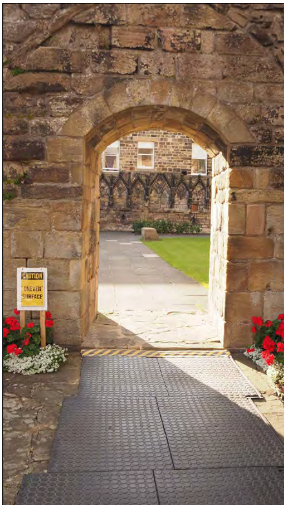
Photo 4. View looking west through an opening in the Calefactory Wall, shown prior to works.
