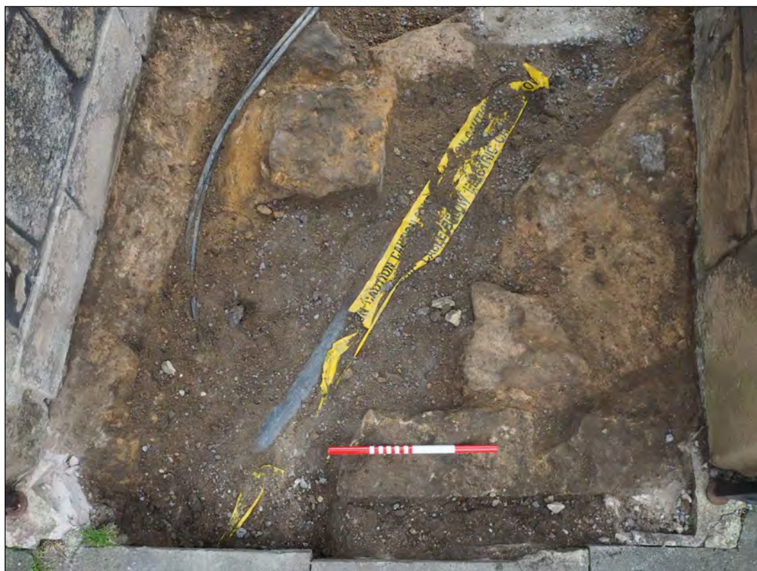
Photo 6. View looking west through an opening in the Calefactory Wall, showing services truncating the wall foundations.
