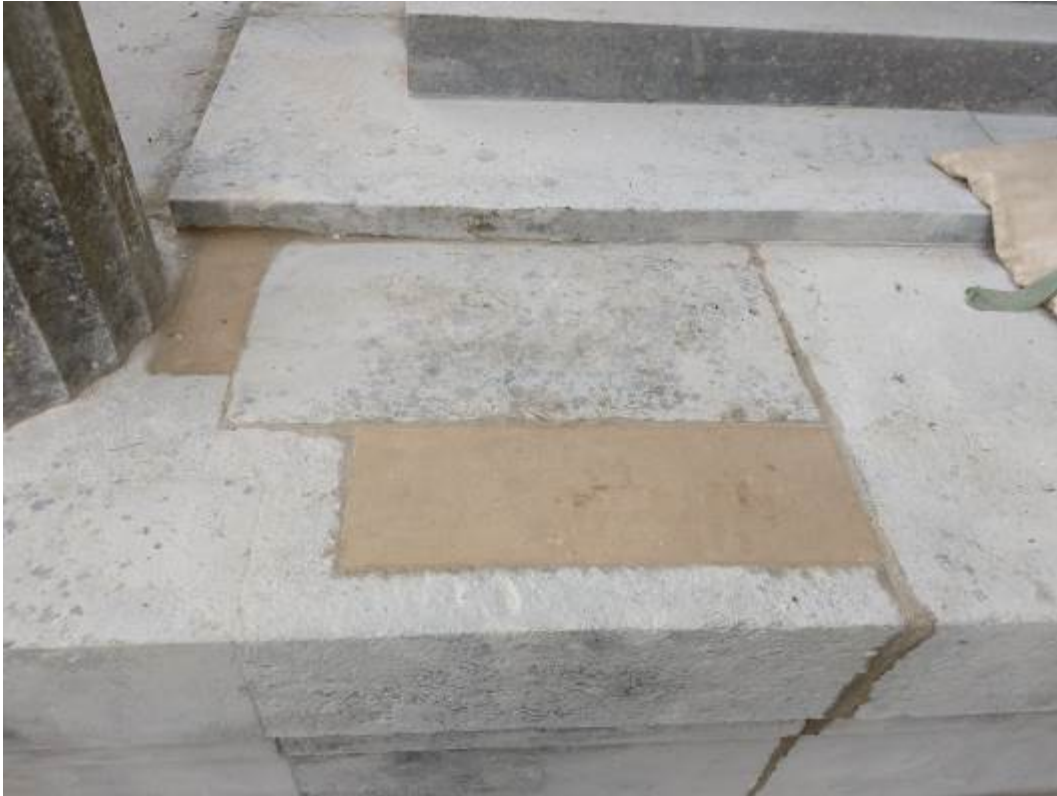
New stone fitted to base of monument
