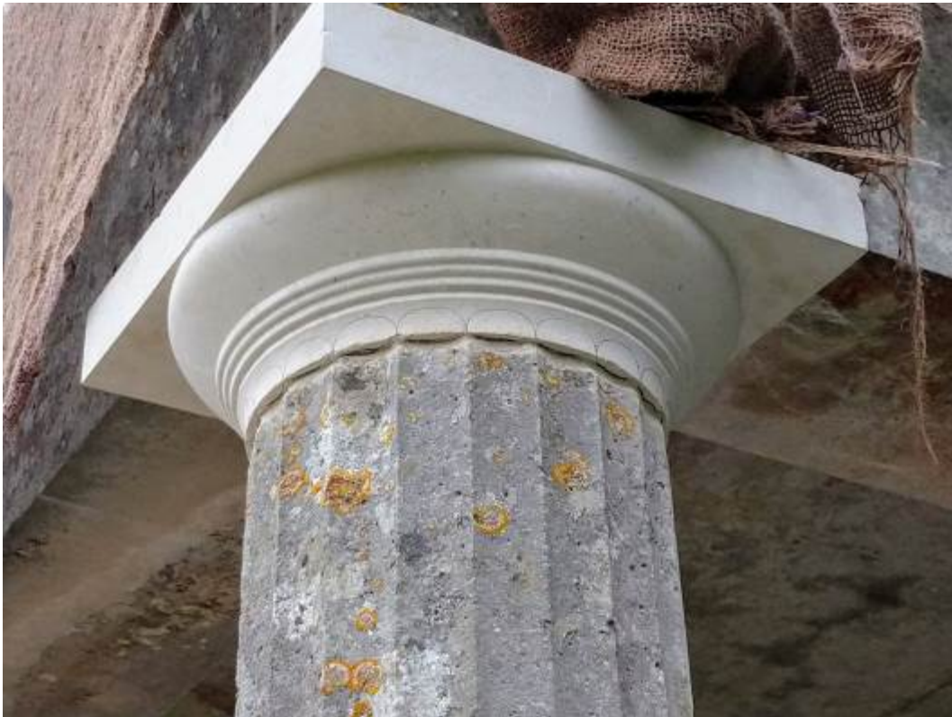
New capital fitted prior to trimming in of flute 'stooling'.
