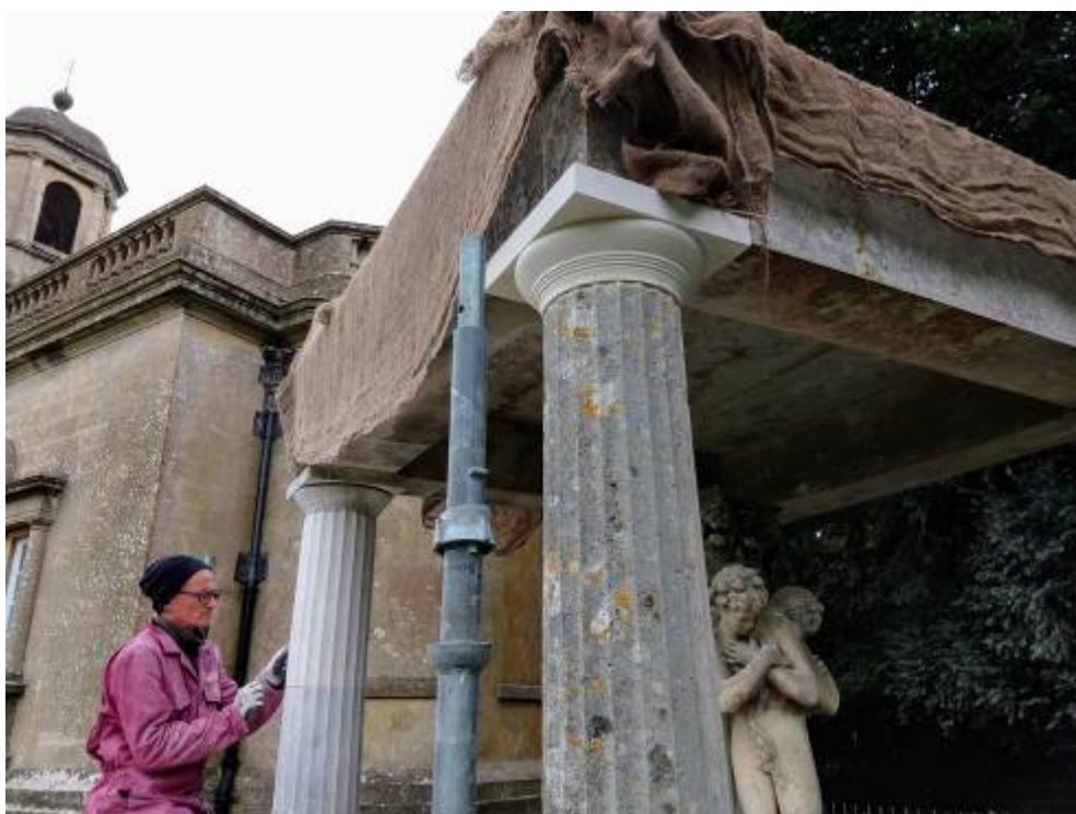
Column section fitted, flutes cut
