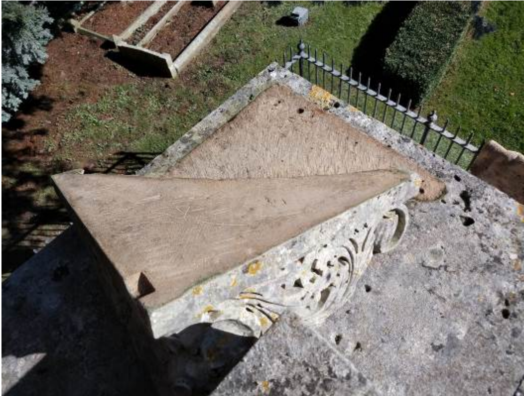
Acroterion lifted prior to re-setting
