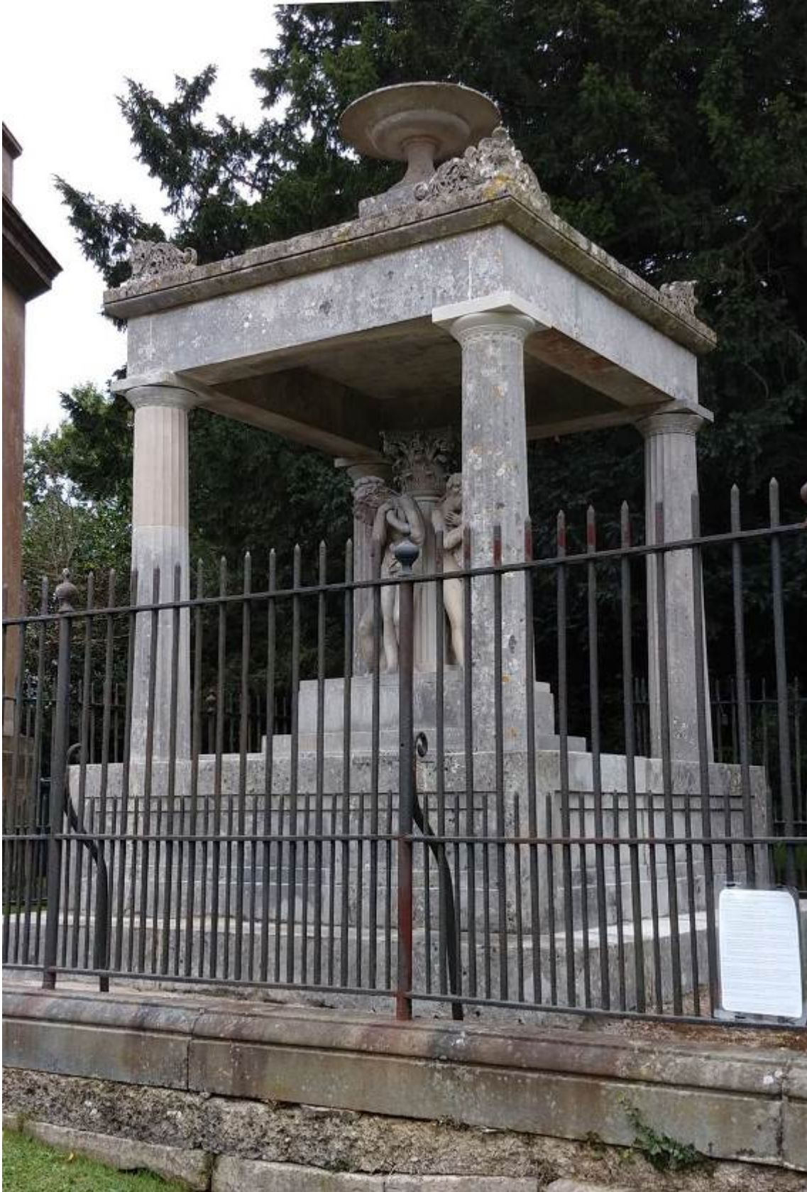
Works to monument completed, new stone trimmed in
