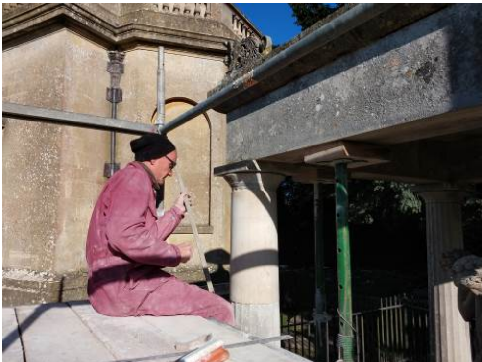
Column section in position, marking up for fluting
