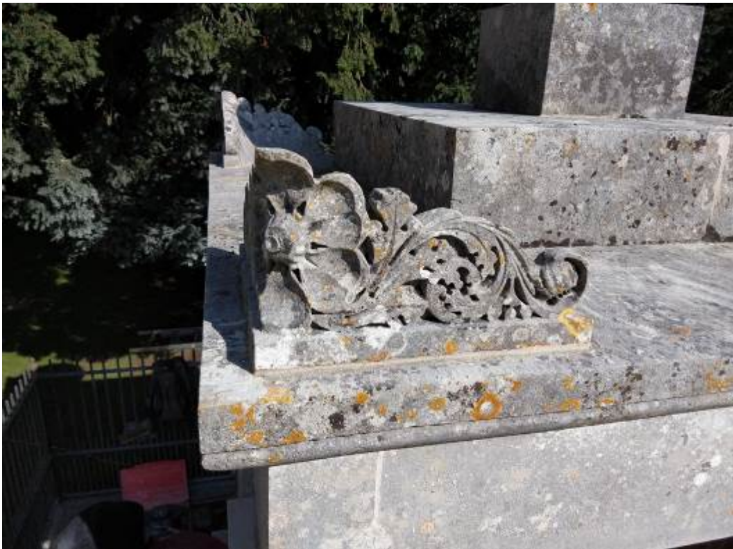
Acroterion re-positioned and bedded
