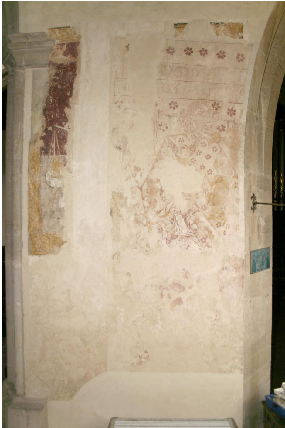
Fig 2. The South aisle, tower pier – overall view (after conservation)
