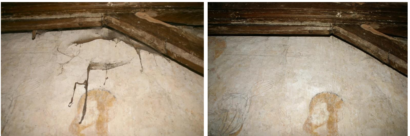
Fig 13. Upper east wall, before and after treatment
