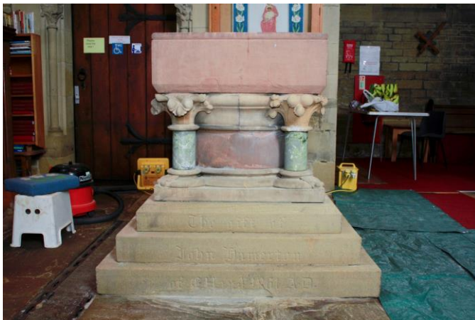
The font after all cleaning processes, note the more obvious difference in colour and texture between the different materials and paving in the foreground.
