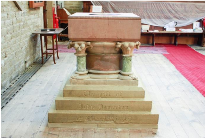
A context view showing the incised inscription to the bottom three courses of the stepped base. Note the lustre on the green marble columnettes which no longer appear dull and lifeless.
