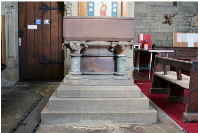
The font before any treatments with the hardwood door, the original entrance into the church, to the left. The font sat in front of the kitchen and welfare facilities.
