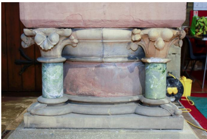
A cleaning contrast showing the right-hand capital and everything above having been cleaned. The vulnerable faces of the font bowl were cleaned with paper-towelling compresses as they were not up-to low-pressure steam cleaning.
