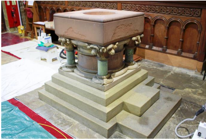
Cleaning in progress, whilst the opening-up works take place in tandem.
