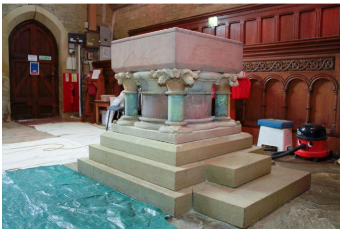
Another view of the font after all cleaning processes. The font received direct (albeit diffused) sun from the tall windows to the south. This would have meant repeated heating and cooling cycles over the decades, perfect for soluble salts in which to flourish. It is shielded from the sun in its new location and its proximity to the nearby south wall.
