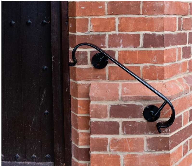
Handrail at rear door
