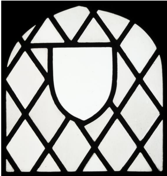
Head panel with laminated glass protection in place of shield
