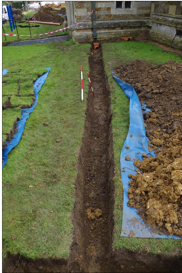
Photo 18. Drain Trench 9 with Soakaway 4 in foreground, looking E.
