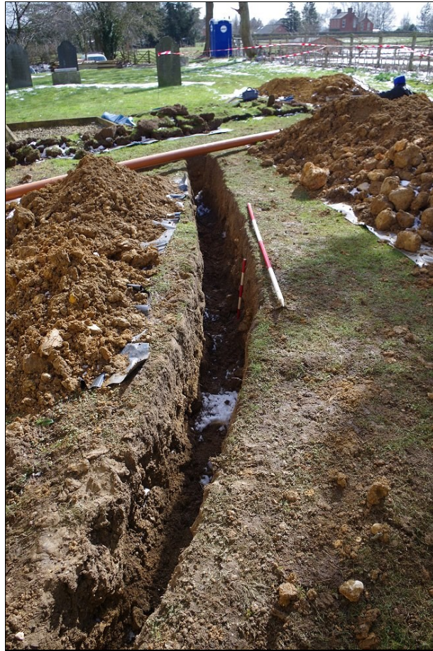
Photo 15. Drain Trench 8, looking SE.
