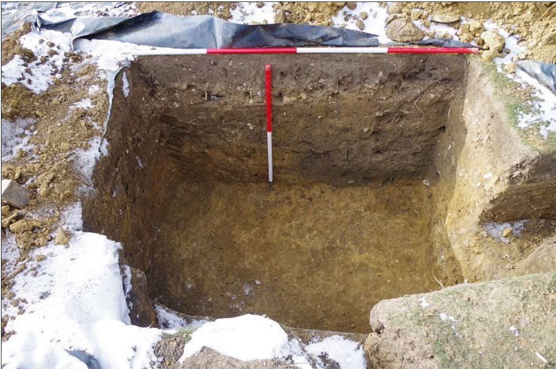
Photo 6. Soakaway 4, looking S (Drain 6 on right of frame).
