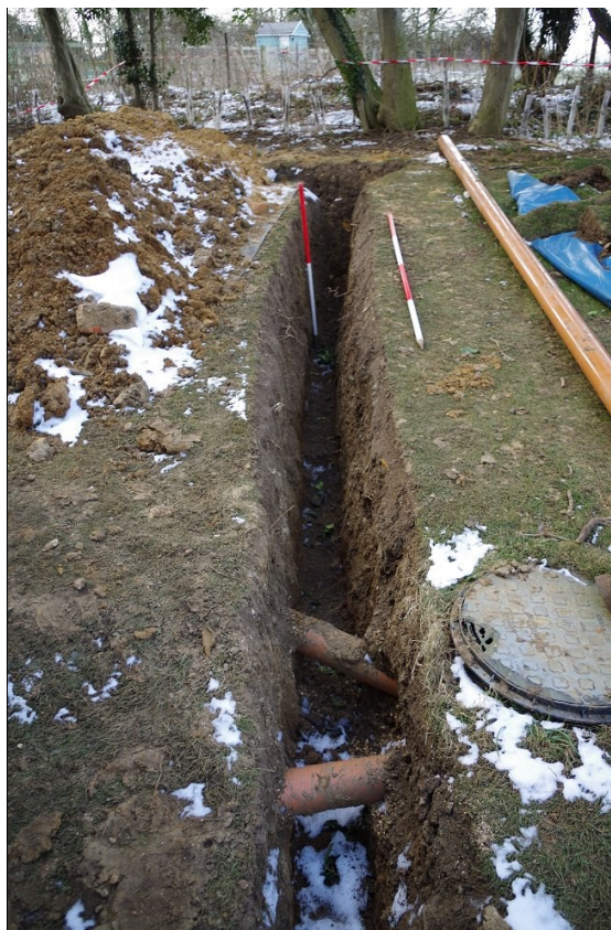
Photo 12. Drain Trench 5, looking SSE towards Soakaway 3.
