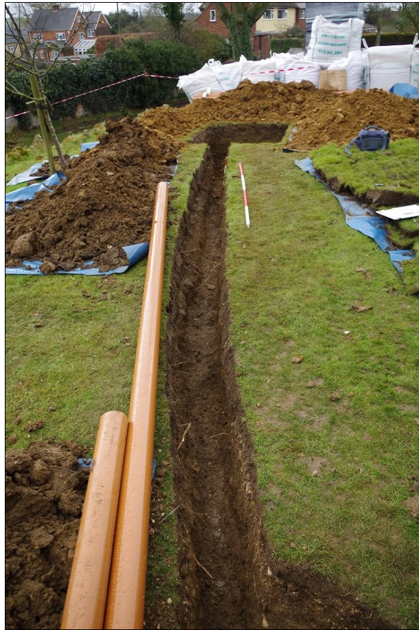
Photo 10. Eastern part of Drain Trench 1 and Soakaway 1, looking E.
