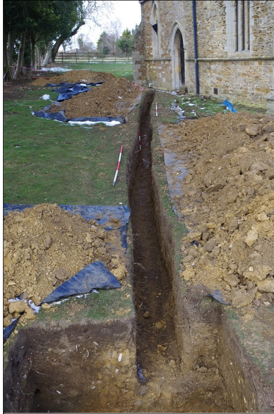
Photo 13. Drain Trench 6 with Soakaway 4 in foreground, looking WNW.
