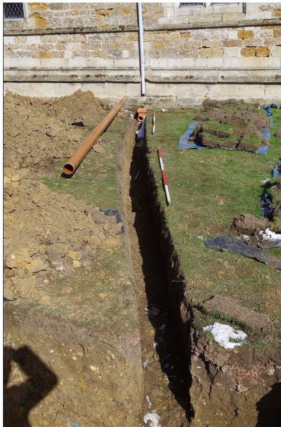
Photo 14. Drain Trench 7, looking NNW.
