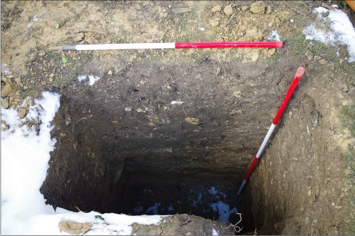
Photo 5. Soakaway 3, looking S.
