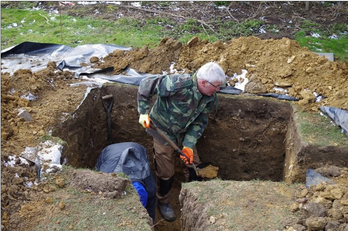
Photo 2. General View of Excavation in Progress (Soakaway 4), looking S.
