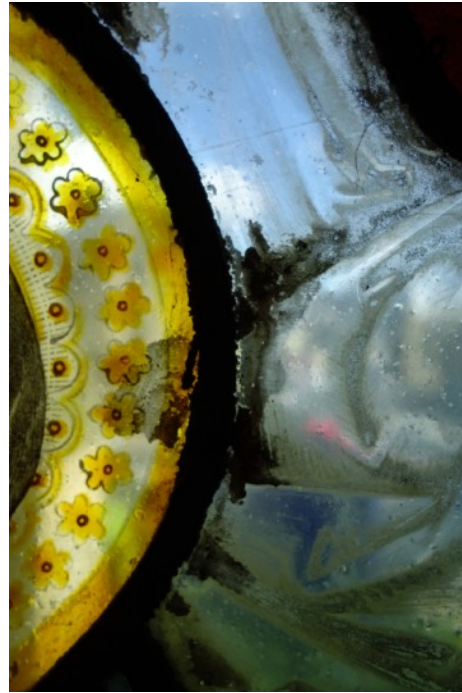
details: unpainted repair/ leached leaded light cement
