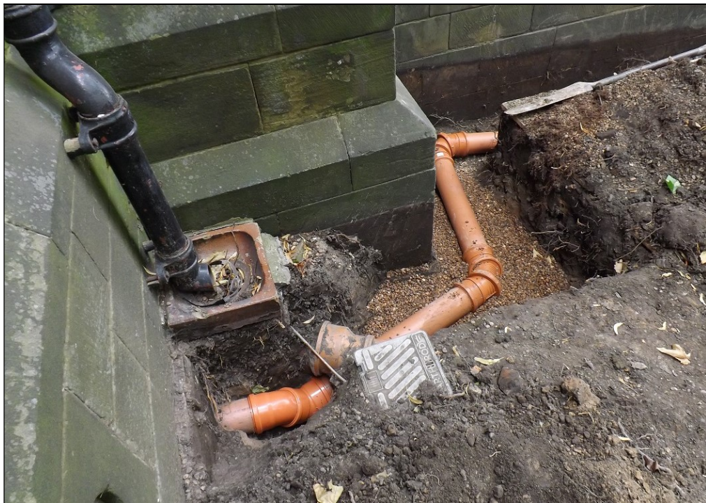
Plate 1. Area of excavation in vestry, looking north-east
