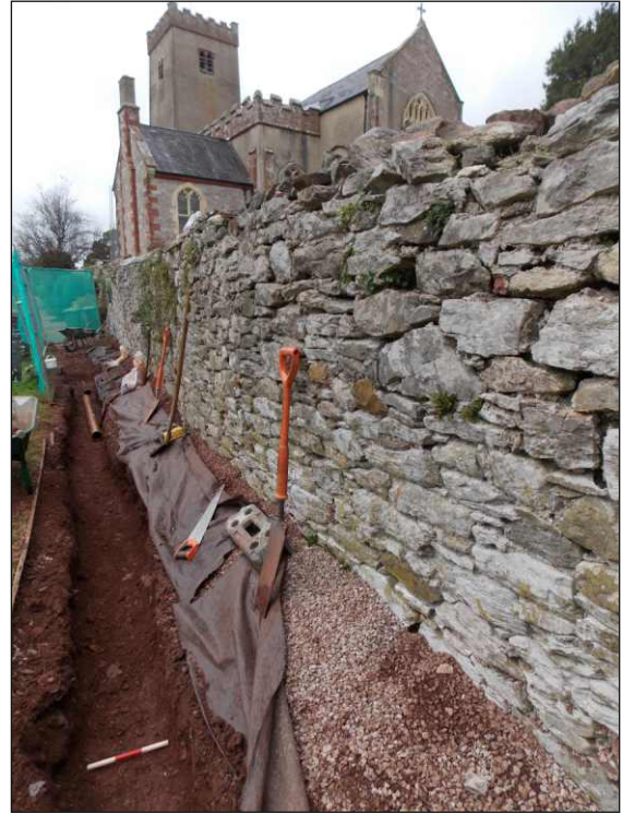
Plate 11: Drainage trench excavation, view to southwest (scale 0.3m)
