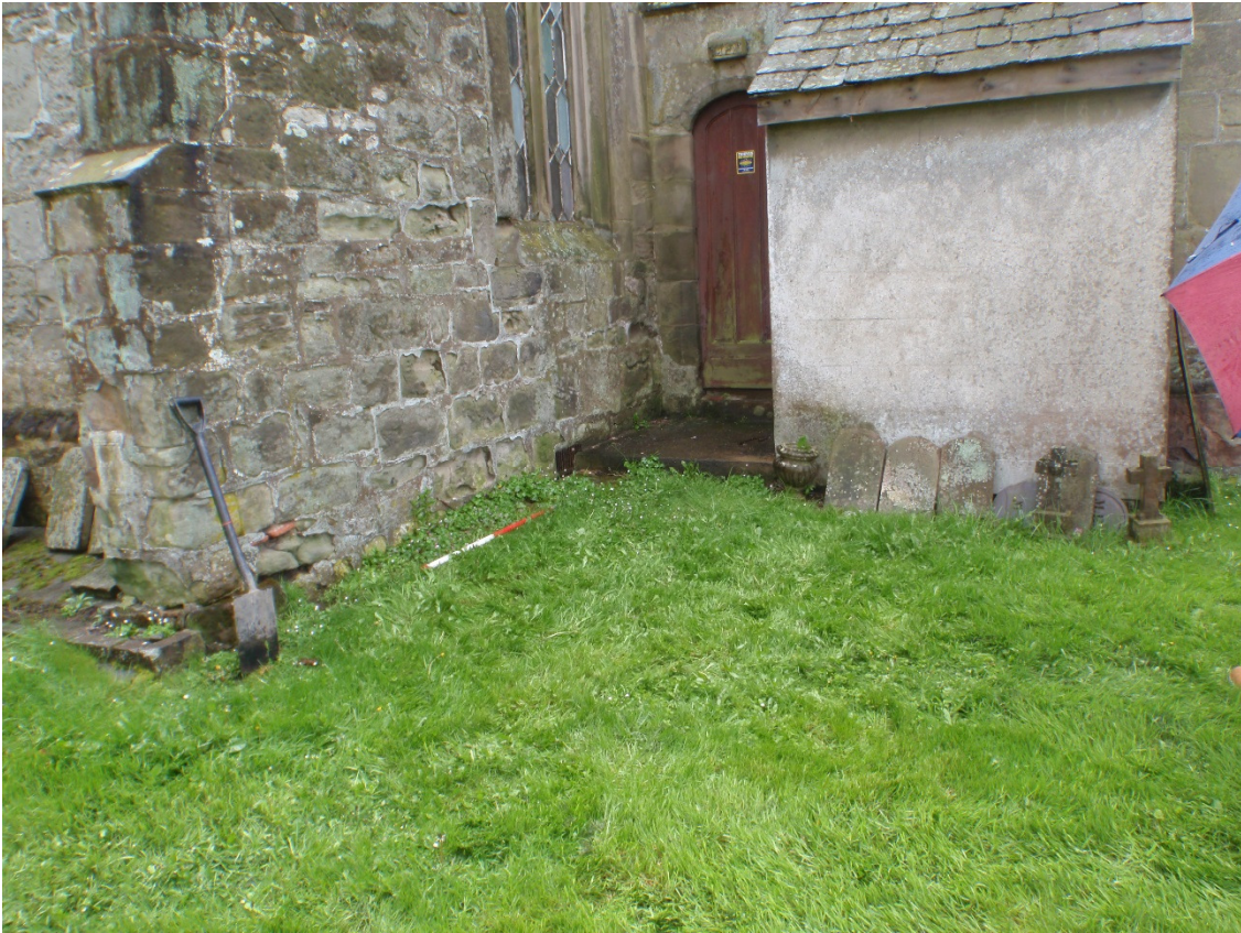
Plate 1. Location of the two test pits prior to excavation looking southeast
