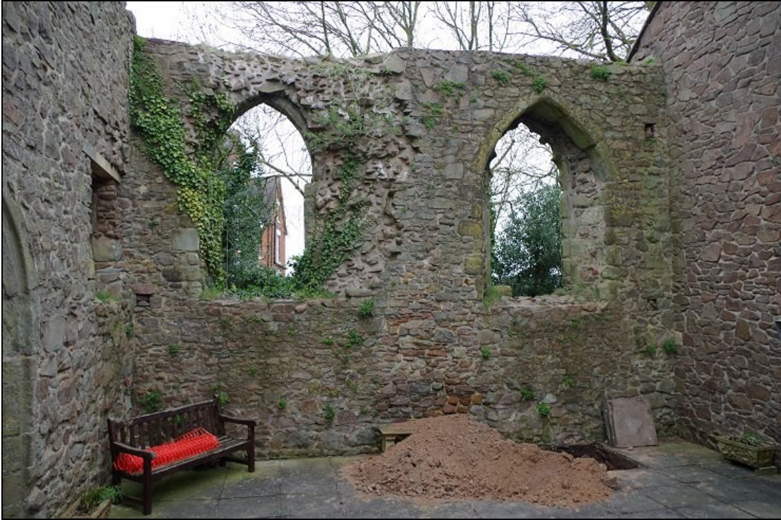
Photo 5. Interior of unroofed part of Nave, looking NNE towards Trial Pit 2.
