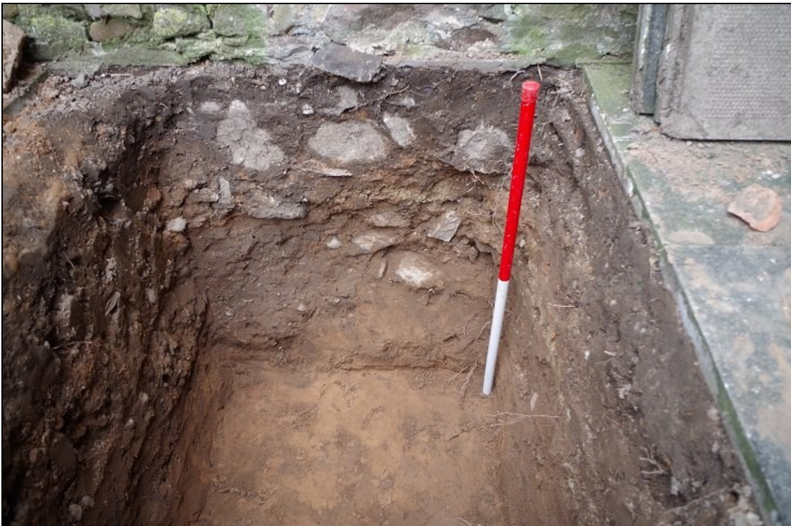
Photo 6. Trial Pit 2 showing north wall of nave (1), looking N.
