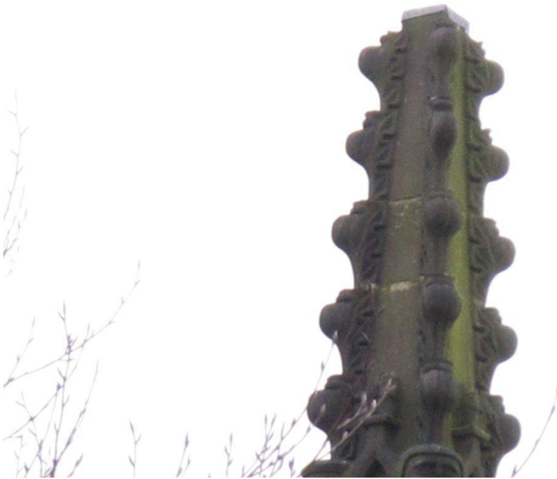
Pinnacle showing new lead cap to protect exposed dowel and masonry
