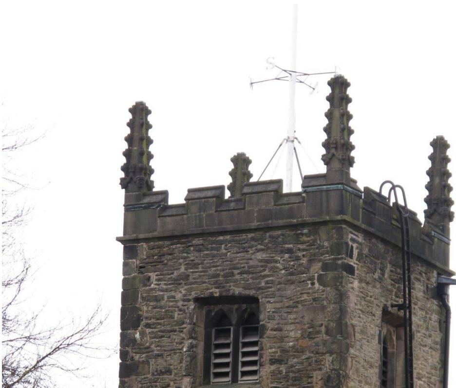
Close up of Tower with all four finials in view
