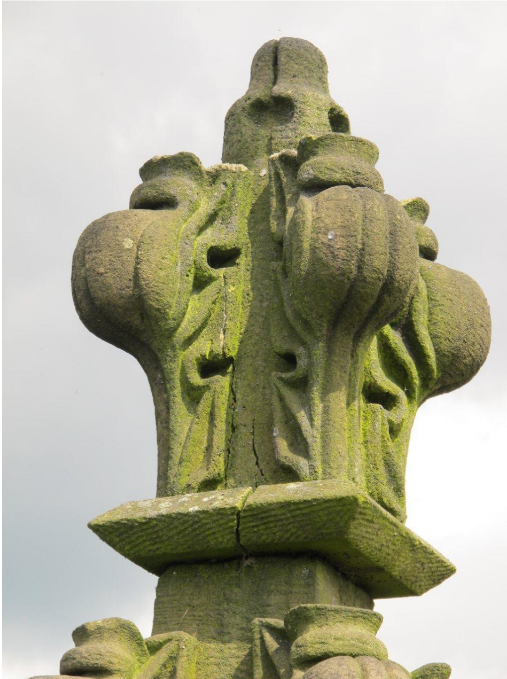
Example of Finial cap – now removed and safely stowed
