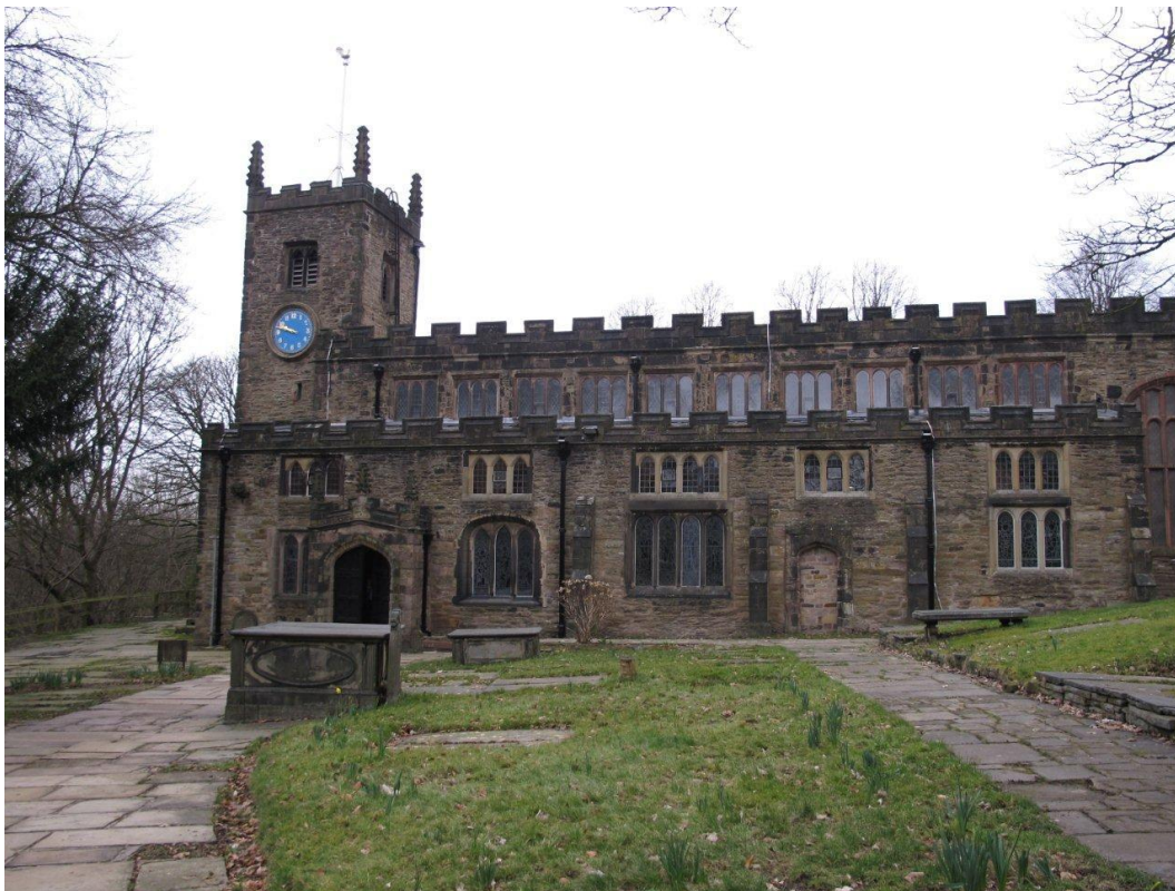
External south elevation showing the pinnacles without their caps
