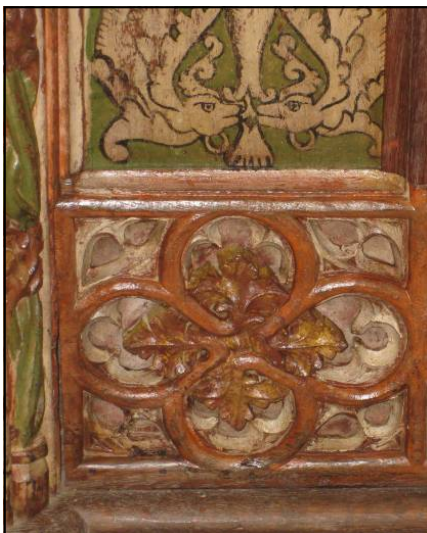
Many bosses and paterae appear to have lost their colour and it is the red ochre primer that is visible. However, careful cleaning reveals many pockets of the golden yellow pigment, orpiment. This problematic pigment, composed of sulphide of arsenic, surprisingly retains its golden colour, when usually it turns brown (see left and above).
