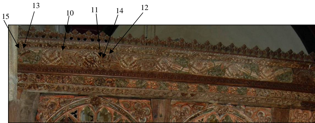
Cornice: Bays 1 and 2
