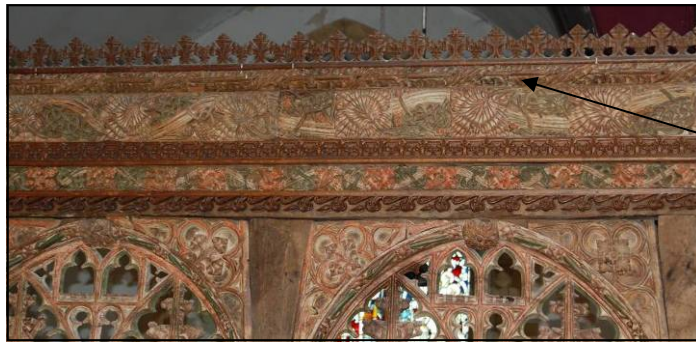
Location of sample 16 taken from Bay 5, south end of screen
