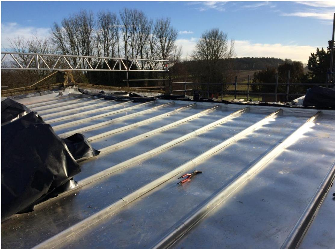
10. Stainless steel roof capping laying underway 19/12/2017
