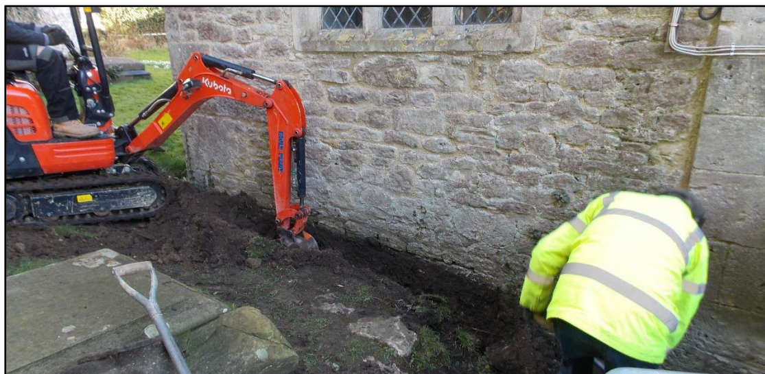
Figure 2. New drainage channel under excavation.
