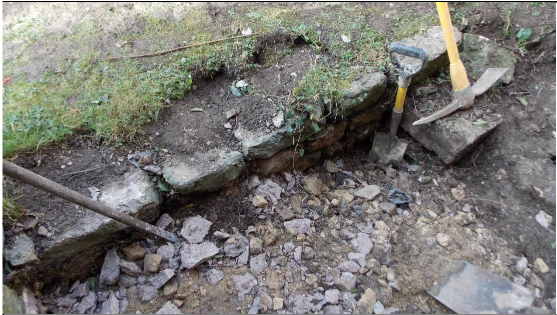
Figure 6. Retaining wall: facing NW.
