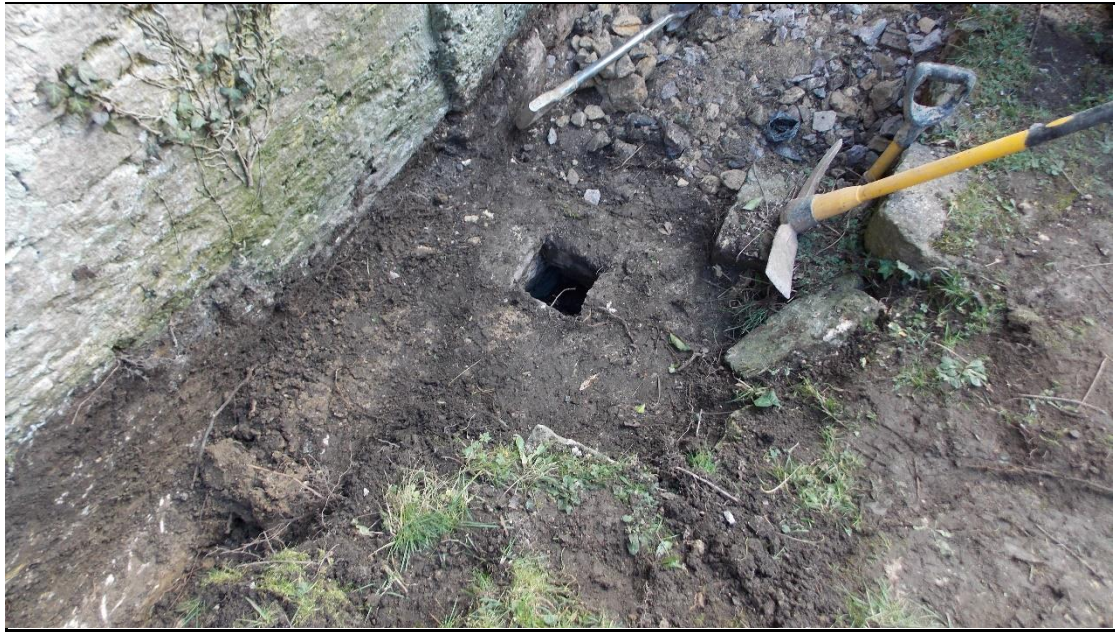
Figure 4. Existing drain: facing SE.
