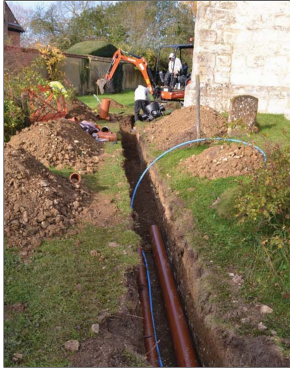
Plate 1. Main pipe trench in west, looking north west.
