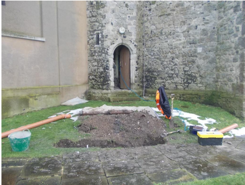
(Fig 3 – excavation trench in the foreground, looking north-west)
