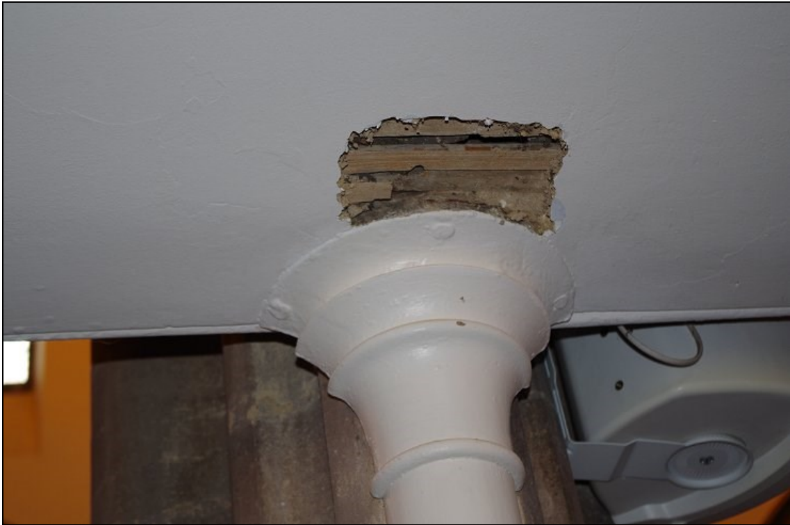
Photo 9. Intervention 5: Plaster removed from ceiling below N gallery, looking S.
