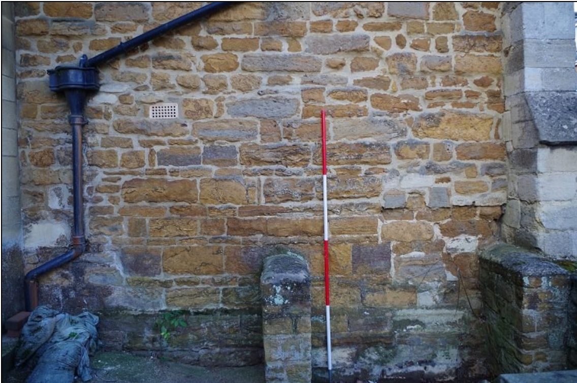
Photo 16. External face of east wall of north porch, looking W.
