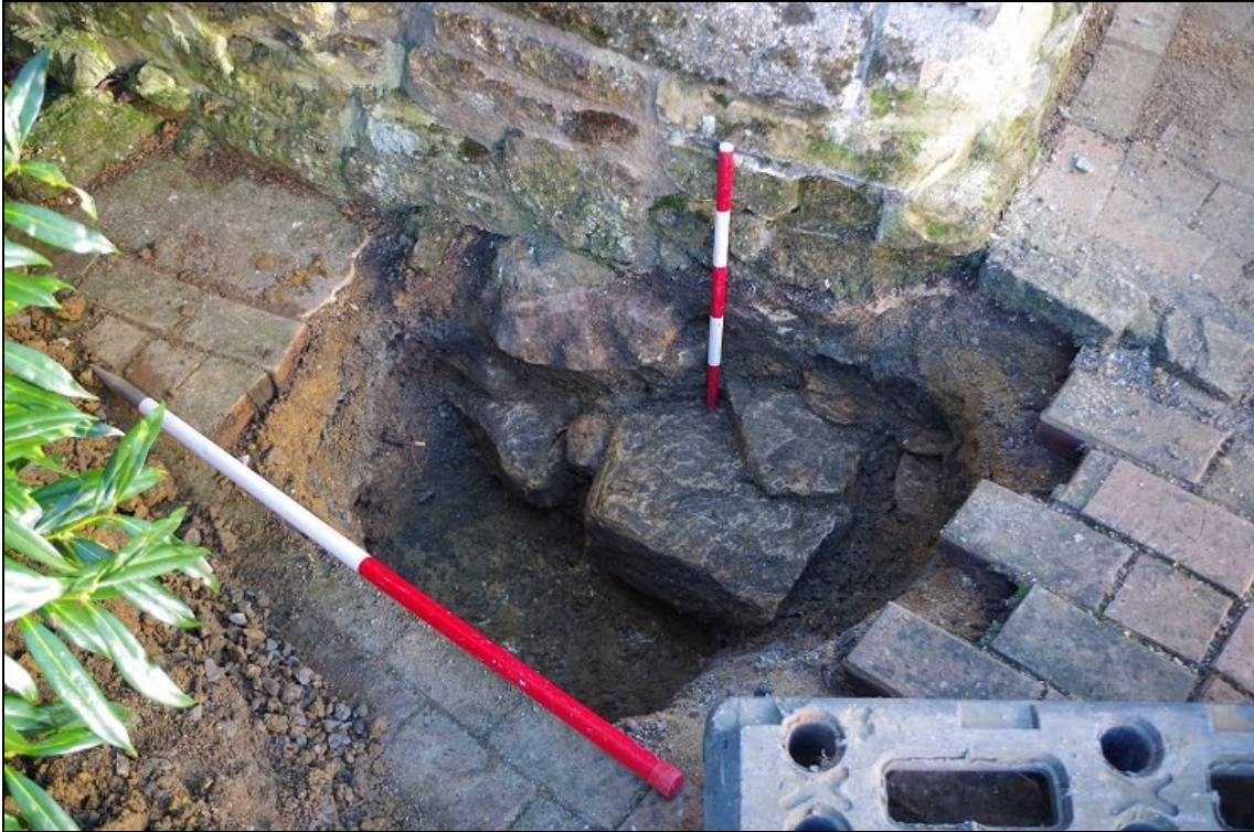
Photo 13. Intervention 8: Footing exposed at north-east corner of north aisle, looking SW.
