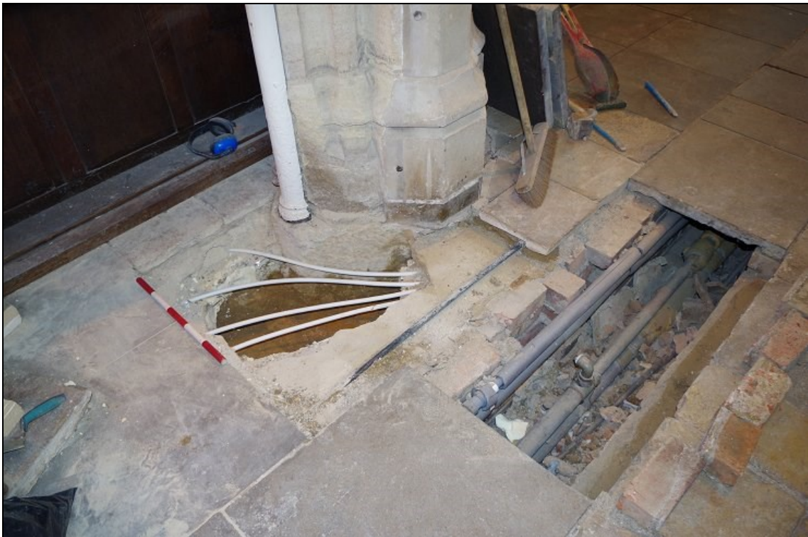
Photo 4. Intervention 1: Showing heating duct & stone footing below pier base, looking SE.
