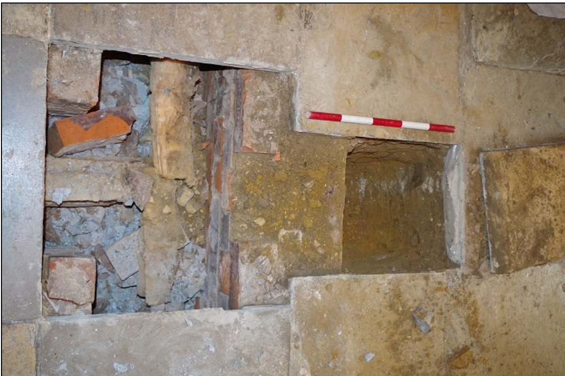
Photo 6. Intervention 2: Heating duct (left) and geological natural ground (right), looking E.
