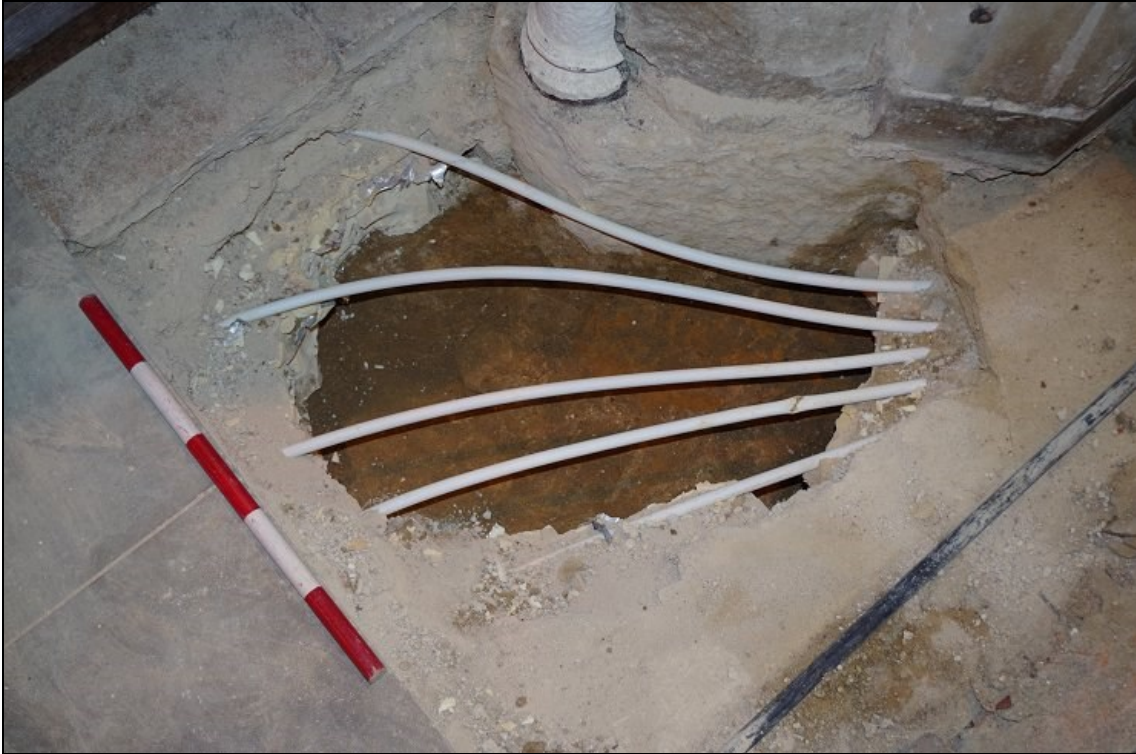
Photo 5. Intervention 1: Detail of mortared ironstone footing below pier base, looking SE.
